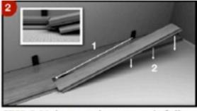
STEP 2:Make sure the tongue is fully inserted into the groove, then drop down the floor.
