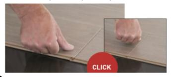
DISENGAGE - long side Start disengaging on the long side by lifting the plank in angle position.
