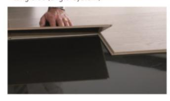
SHORT SIDE To engage on the short side, let the plank drop easily.
